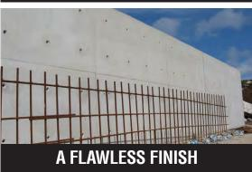
Nox-Crete's Release Agent #10 (RA #10) reacts chemically with the alkalies in concrete to form a soapy film which allows trapped air and excess water to escape during vibration, minimizing surface voids and providing a smooth, uniform concrete finish.
