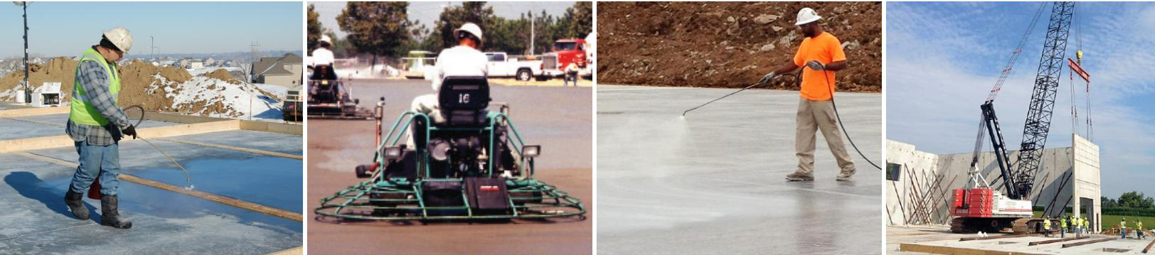
ASTM C309 has long been the standard by which membrane-forming concrete curing compounds are judged.
