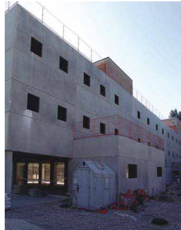
Industrial building with precasted panels
