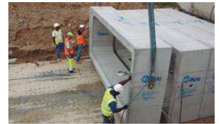
Installation of finish product
