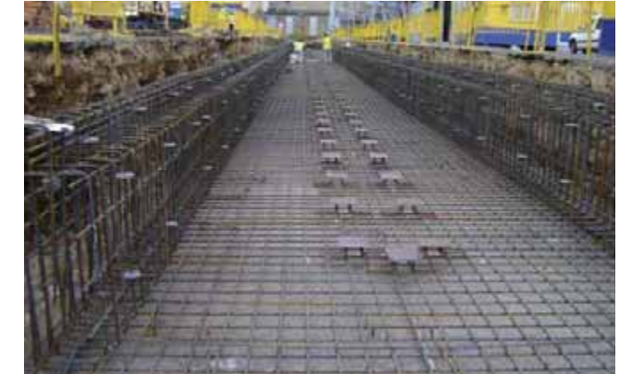
Production of bridge girder on a concrete bed
