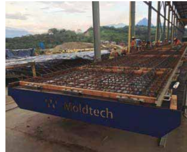
Fixed table for pre-slab
