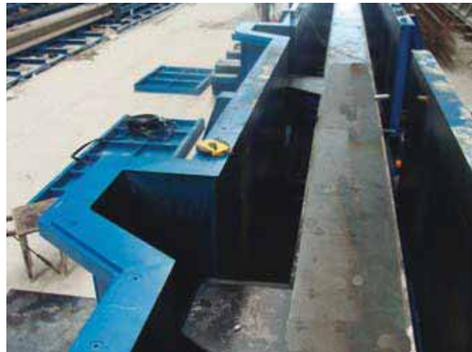
Detail of corbel shape
