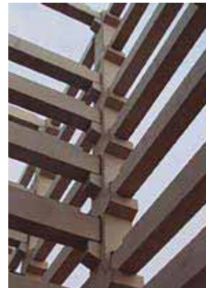
Example of column with a large amount of corbels
