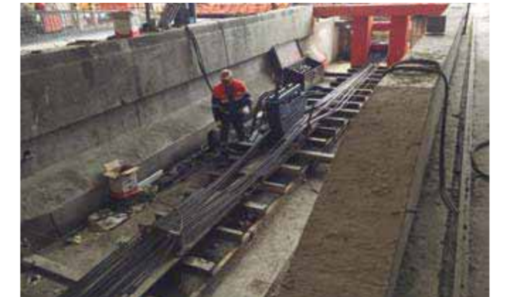
Construction of the concrete reactioning structure
