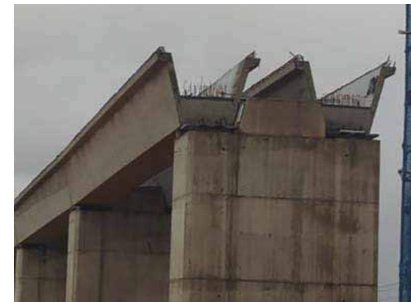
Shuttering with protruding bars
