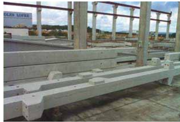
Columns with 2 corbels
