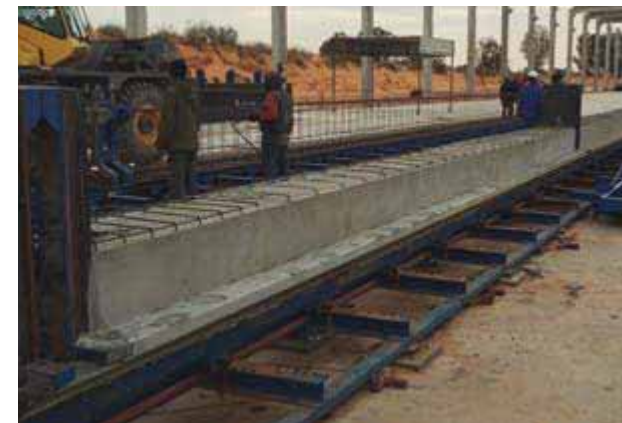
Production on casting bed
