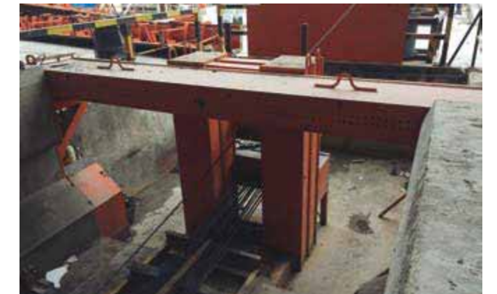
Passive stressing head on self-supporting bed
