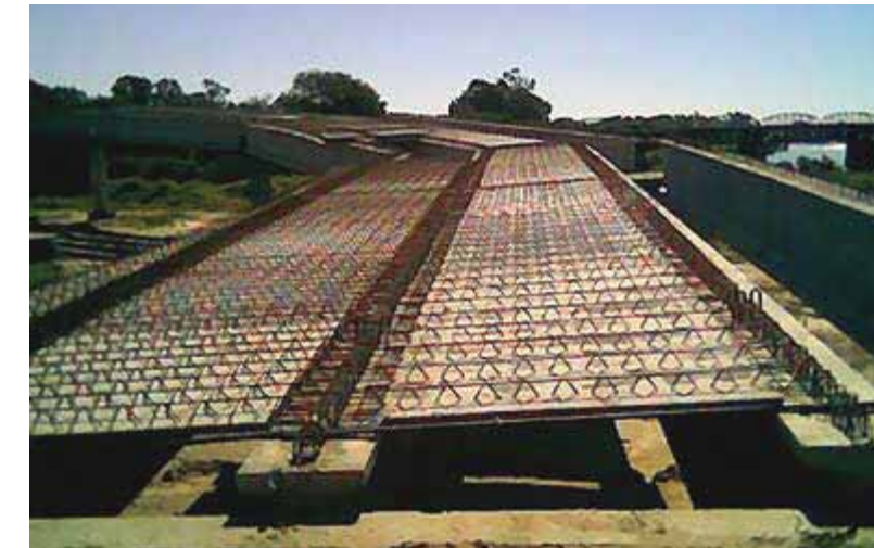
Making a slab with pre-slabs in a viaduct
