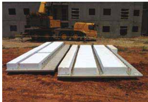
Example of pre-slab for residential floor
