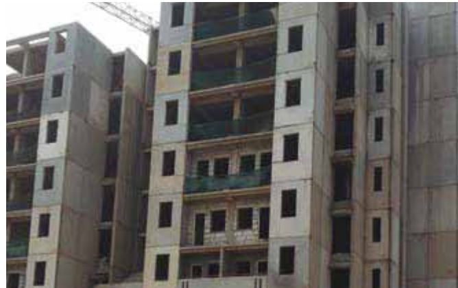
India: building construction with precasted elements
