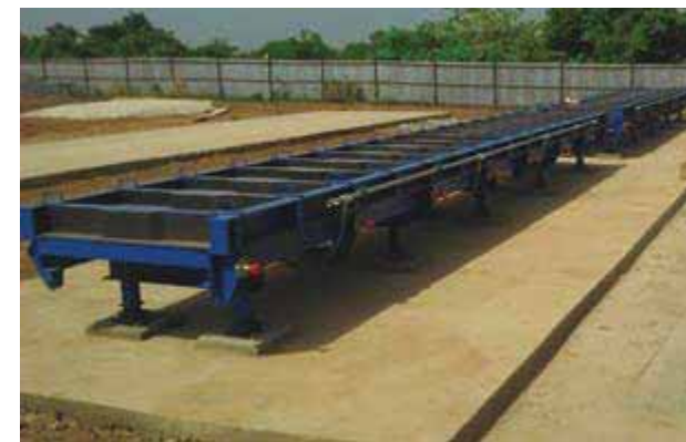
Fixed table for making drainage channel covers
