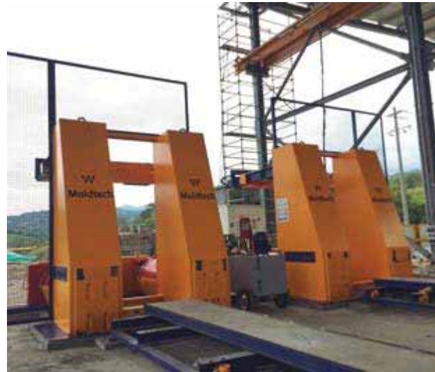
Casting bed for pre-stressed elements
