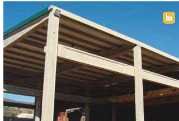
'I' beam as part of a building structure
