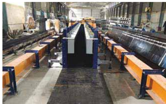
Production of inverted T beam on a concrete bed
