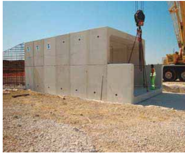
Placement of half frame as highway underpass
