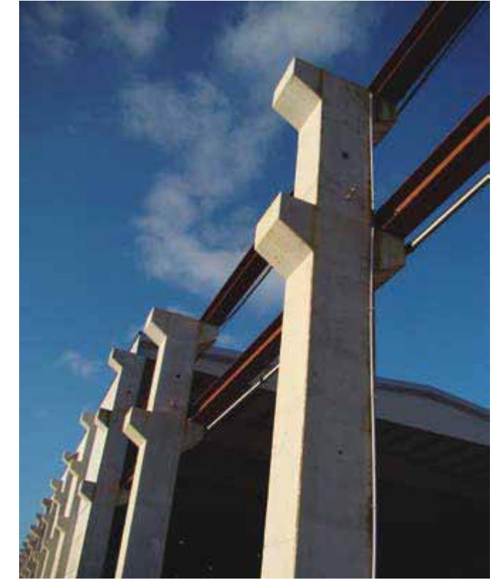
Precast columns with corbels
