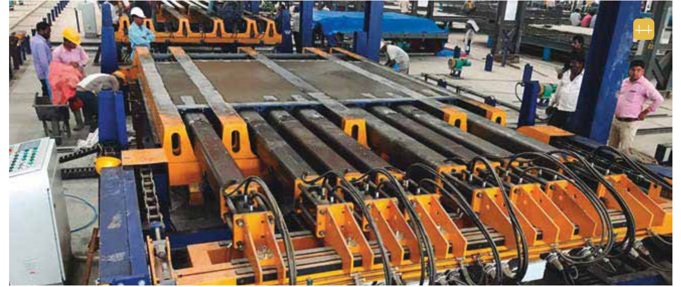
Moulds ready for demoulding
