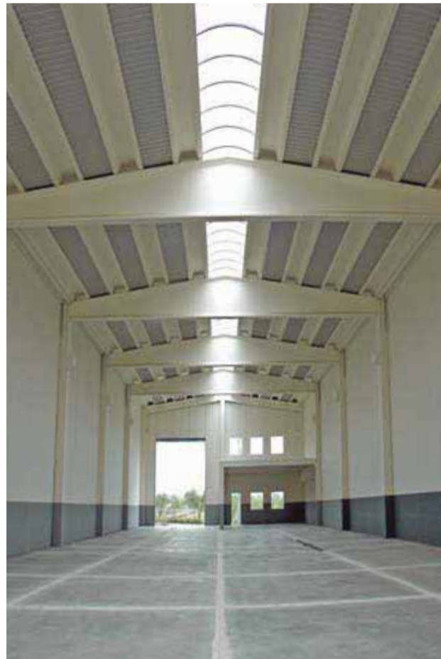
Industrial building with delta beam and roof beam
