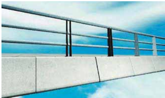
Detail of bridge wings
