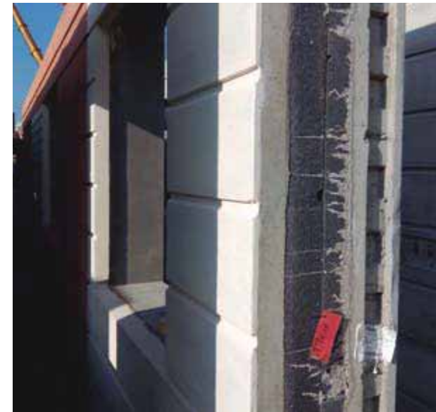
Detail of residential panel with insulation
