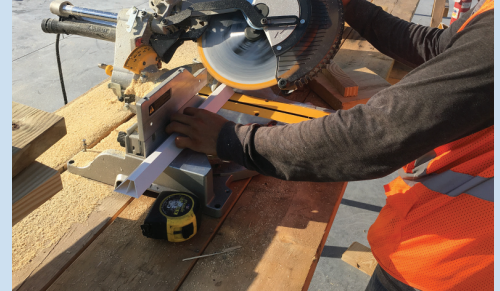
Cut Clean Line Reveal Strips to the desired size using a miter saw.
