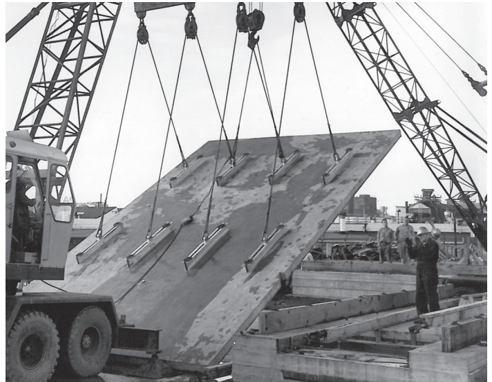
NOX-CRETE BONDBREAKER USED ON CIRCA 1964 TILT-UP PROJECT
