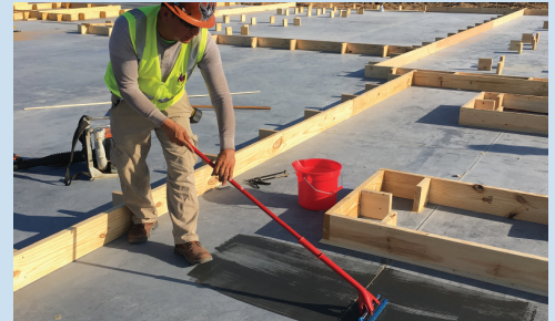
Thoroughly clean area with alcohol or similar cleaner before gluing down.
