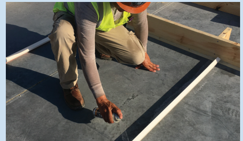
Using construction adhesive, glue Clean Line Reveal Strips into place.
