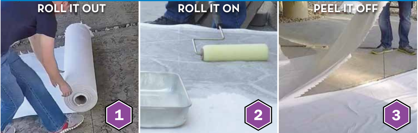
SAFELY AND EFFECTIVELY REJUVENATE OR STRIP OFF OLD, WORN-OUT DECORATIVE ACRYLIC SEALERS
