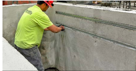
EXCELLENT PRECAST USES
