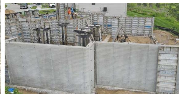
PRO-RELEASE 3.0 is a cost-effective, water-based concrete form release agent designed for superior performance across a wide range of concrete mix designs. Combining both chemically active and barrier-type components, PRO-RELEASE 3.0 ensures easy form release, reduces surface imperfections, and enhances overall results on every project.
