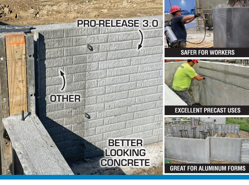
PRO-RELEASE 3.0 is a cost-effective, water-based concrete form release agent designed for superior performance across a wide range of concrete mix designs. Combining both chemically active and barrier-type components, PRO-RELEASE 3.0 ensures easy form release, reduces surface imperfections, and enhances overall results on every project.
