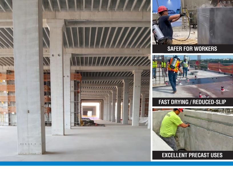
Release Agent #10 E is a revolutionary water-based form release agent designed for use on dense, non-absorptive form surfaces. Its low-viscosity, chemically active formulation allows for application at very light coverage rates, reducing overall costs.
