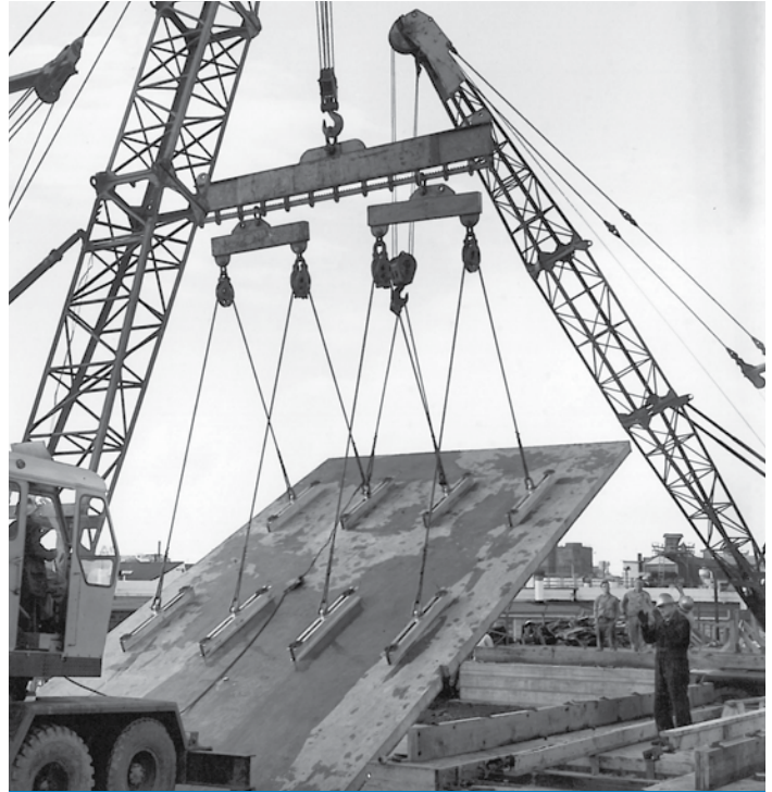
NOX-CRETE BONDBREAKER USED ON CIRCA 1964 TILT-UP PROJECT
