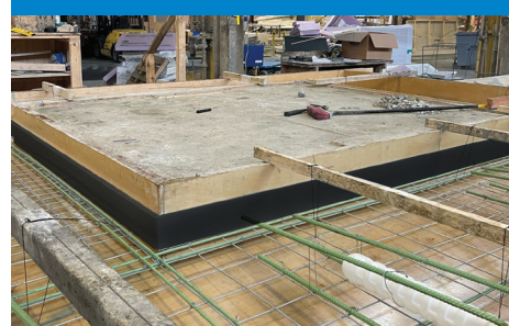
CONCRETE FLOWS INTO THE GROOVE SECURING TIGERLOC PLUS TO THE PANEL
