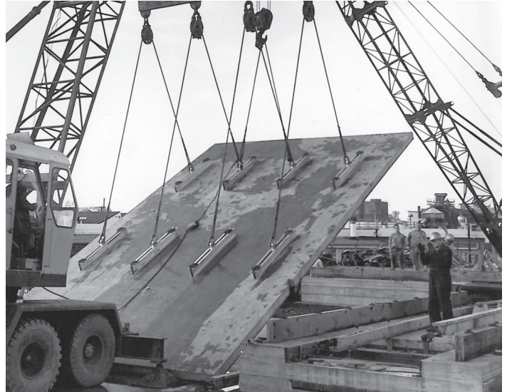
NOX-CRETE BONDBREAKER USED ON CIRCA 1964 TILT-UP PROJECT
